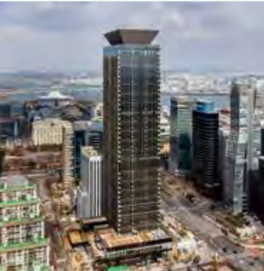
TP Tower Developed a rooftop green park and lower-floor lounge areas for tenants and the community.
