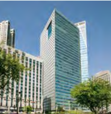
East Central Tower Operated pop-up stores for tenants and provided outdoor rest areas for the local community.
